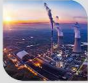
Environmentally friendly heating
