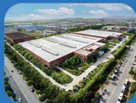
Laishan Industrial Park
