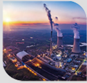
Environmentally friendly heating
