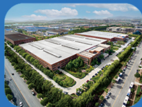
Laishan Industrial Park
